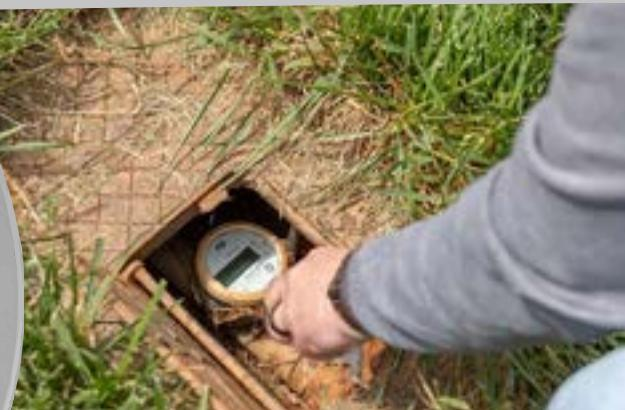
KAMSTRUP Smart Meters are installed outside of your residence or facility. They can aid you in detecting possible water leaks. After checking for leaks on common areas like toilets and faucets, use the meter codes below to identify potential issues.
